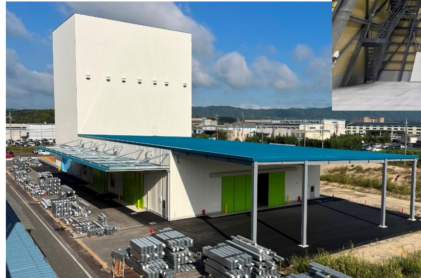
New warehouse and experiment building
